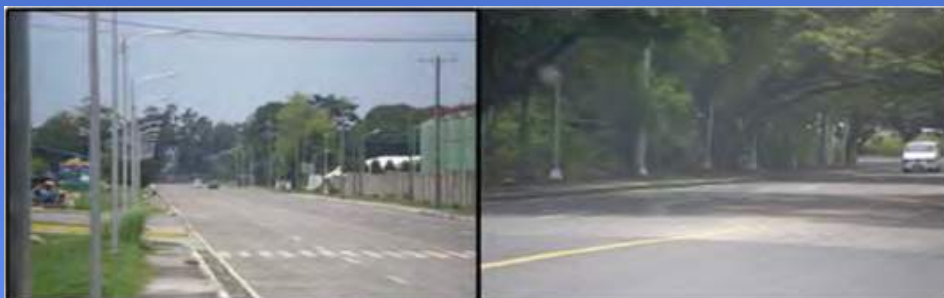
Supply, Delivery, Installation, Testing and Commissioning of SMBA Street lighting Project
