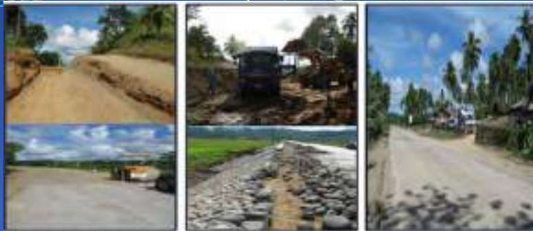
Concreting of Surigao-Davao Coastal Road Cortes-Tandag-Marihatag Road Surigao Del Sur
