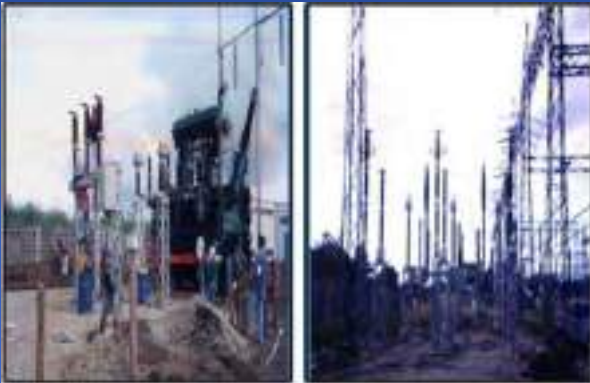
Bacnotan Steel Industries Inc. Calaca 50MVA Substation and Switchyard Expansion
