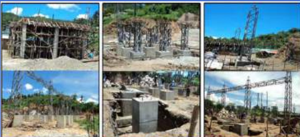
Construction and Installation of 69kV Mobo Substation Mobo, Masbate
