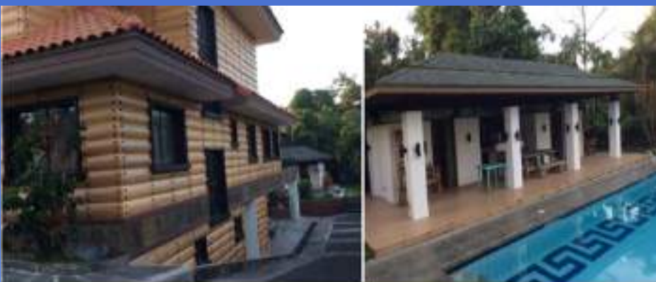
Construction of Private Resorts and Facilities in Amadeo Cavite
