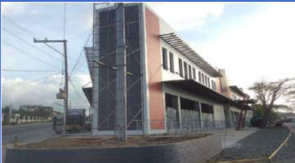
Construction of Paseo Amadeo Mall in Amadeo Cavite
