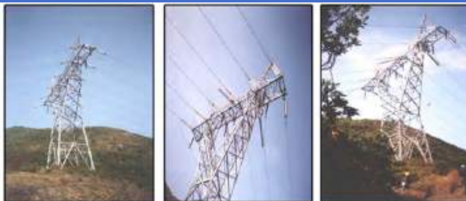
Hong Kong Electric 132kV Line Swapping Project
