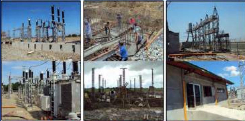
Construction and Installation of 69kV San Jose Substation San Jose, Occidental Mindoro
