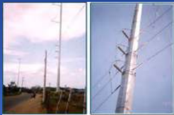
Contruction and Erection of Bacnotan Steel Industries, Inc. 230kV Transmission Line
