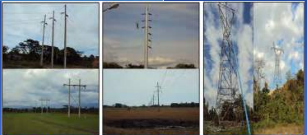
Erection and Installation of Sta. Cruz-San Jose "3" & "4" 69kV Transmission Line Sta. Cruz - San Jose, Occidental Mindoro
