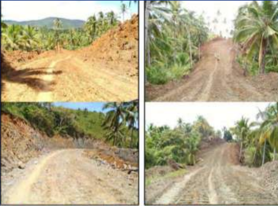
Rehabilitation of Nangka-Bahi Farm-To-Market Road Barobo, Surigao Del Sur
