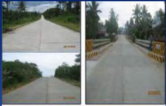
Concreting of Surigao-Davao Coastal Road Hinatuan-Bislig-Boston Section Surigao Del Sur
