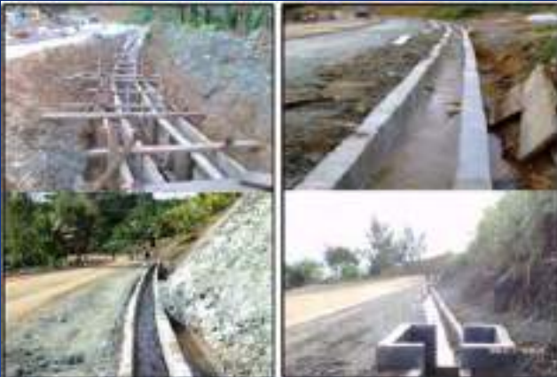
Removal of Slide and Repair of Roads/Pavement Dinagat-Loreto Road
